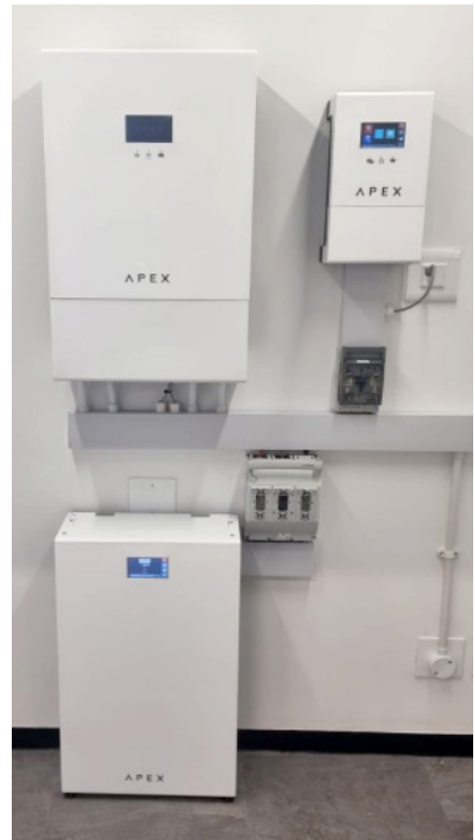
Figure 3. B12K Typical Installation, Connected With A Fuse Disconnecter
